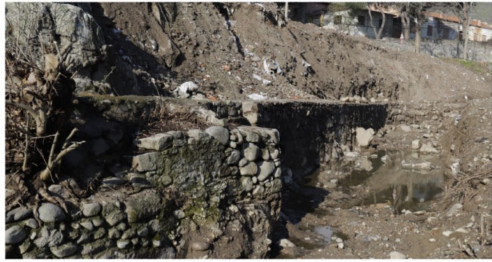
(b) River bank stabilization walls
